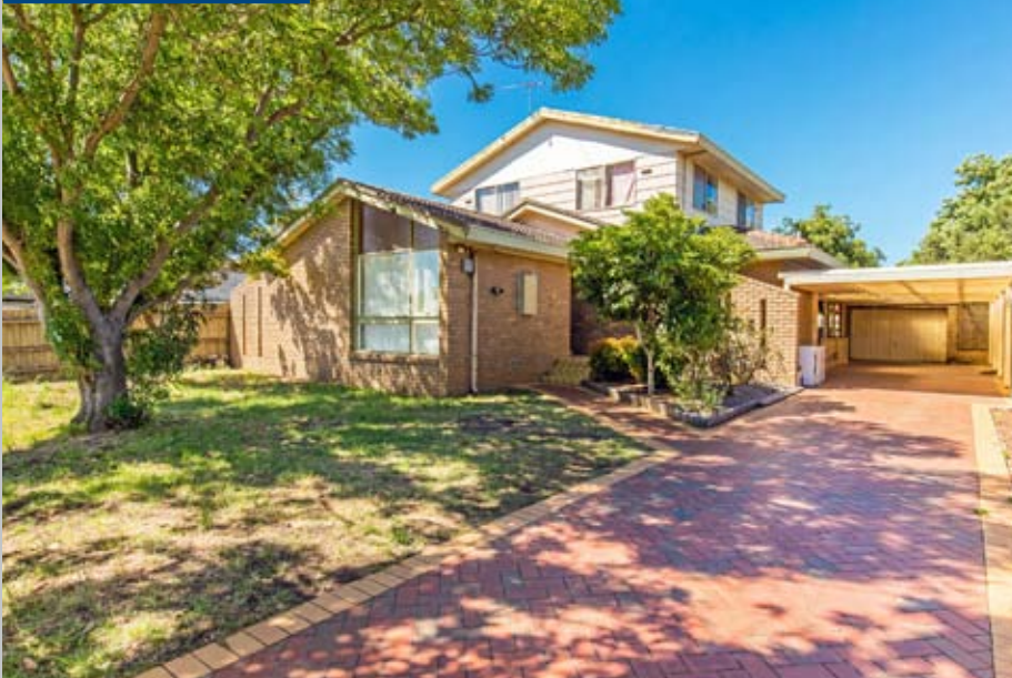
WYNDHAM VALE 5 CASCADE DRIVE
